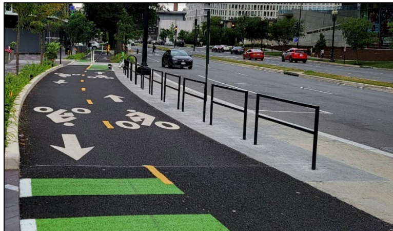
Image of new trail adjacent to Maine Avenue SW
